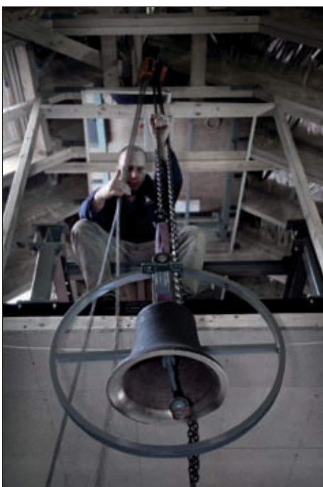
Matthew Higby installing the new tenor at Frosterley
