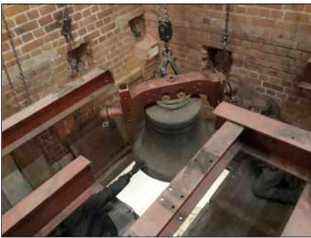
The old tenor on its way down
