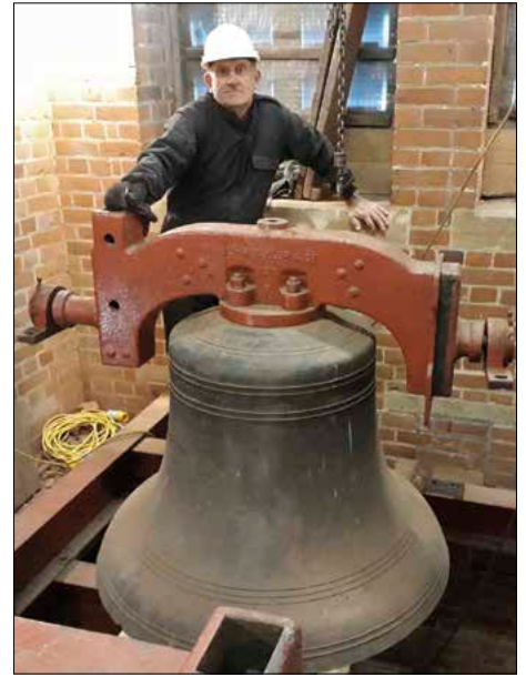
Andy Day with the old tenor waiting to be hoisted down
