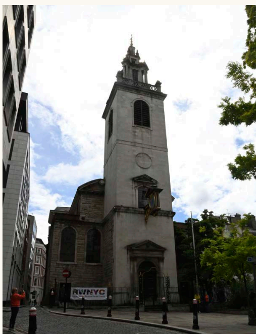
Team photographs by Richard Smith, Iain Anderson and Jonathan Cresshull
